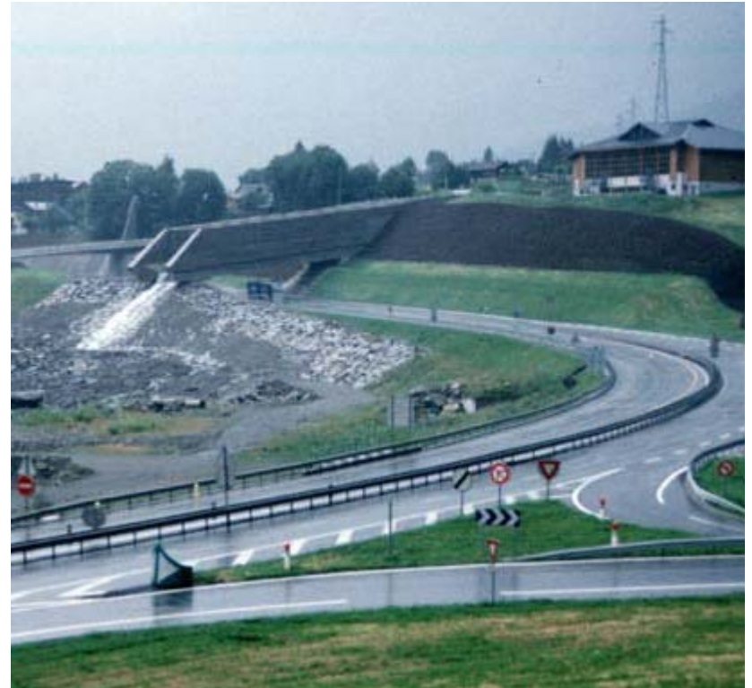
Debris flow bridge in the Savoy Alps, France (Source: the Earth Physics Institute, the University Paris Diderot)
