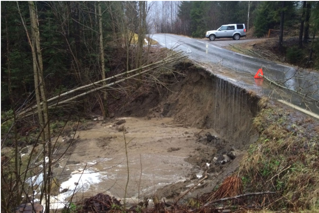
Figure 5-9: Landslide at Hedrumveien in Larvik, 24.12.2013 (Østlands-Posten, photographer: Knut Utklev).
