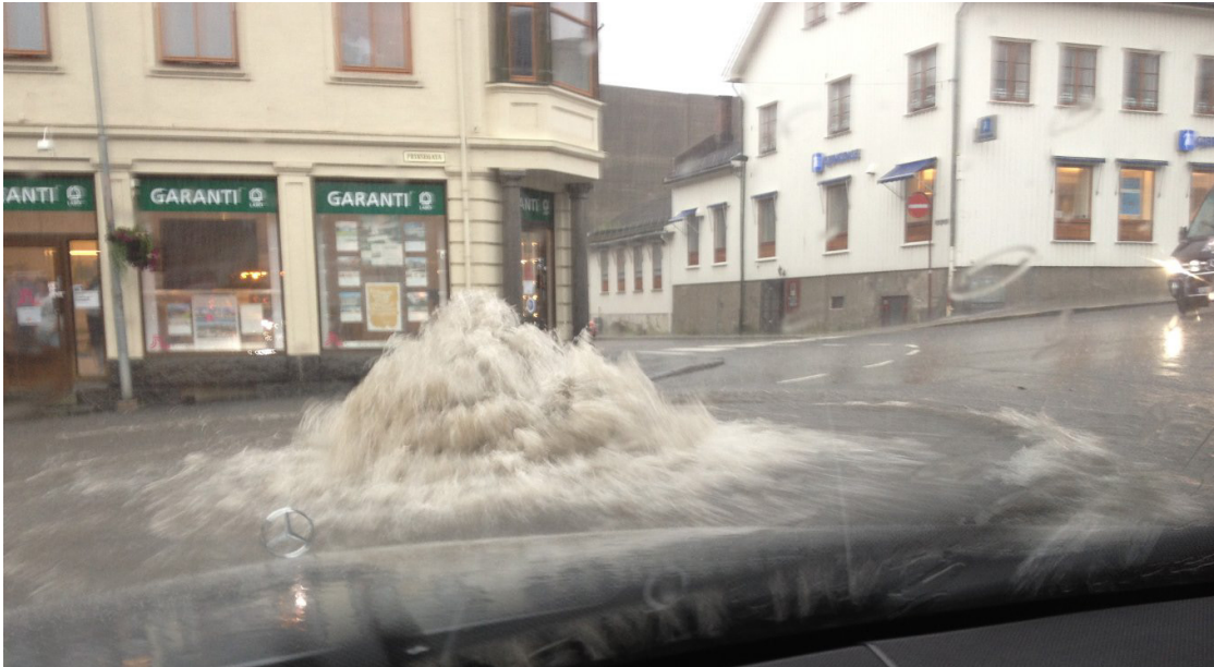
Figure 2-1: Rain water drain in Larvik, exceeding its capacity during a precipitation event on June 29, 2012 ( Østlands-Posten , photographer: Franck Løreng).
