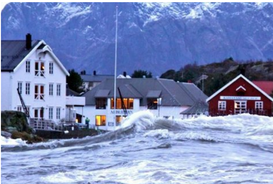
Figure 5-4: Storm surge in Kabelvåg during extreme weather event "Berit", november 2011 (Lofotposten, photographer: Jan Ivar Rødli, Promo Norge).
