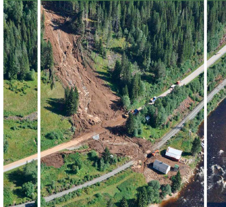
Rainfall-triggered landslides in Almåskroken, 13.08.2013 Photo: Ole Jergen Kjellmark taken from helicopter
