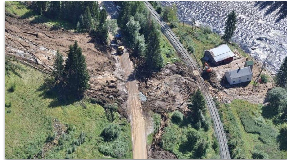
Road cleared after debris flow in Almåskroken, Gaudalen, taken from helicopter shortly after the event (Adressa.no).
